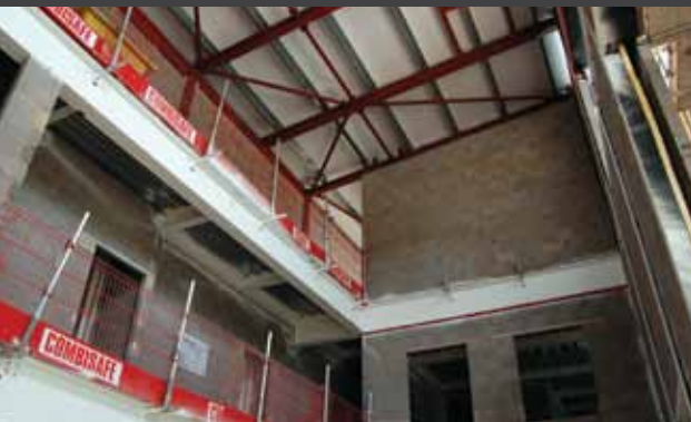
Interior photo under construction
